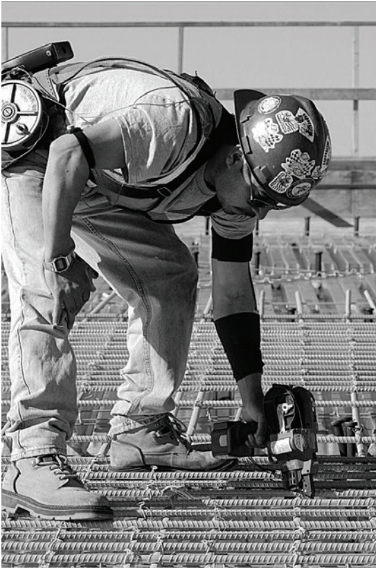
Figure 2. Tying rebar with power tier (PT).
