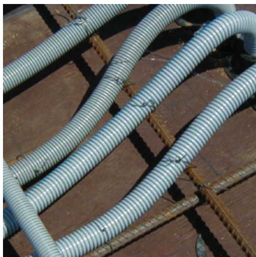
Figure 20: Electrical conduit installed next to rebar steels.
