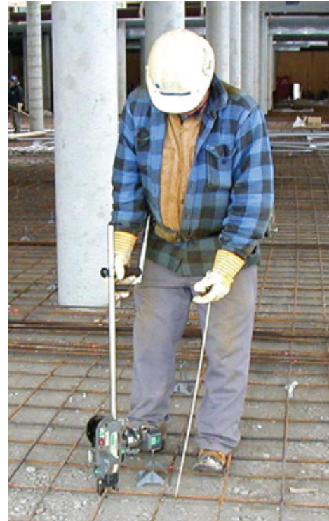
Figure 6: MAX RE-BAR-TIER with arm extension (top) and U-TIER with body extension (bottom). Sometimes a metal hook is used to pull the rebar off the ground so that the wire can be wrapped around the rebar without striking the ground (see top photo).
