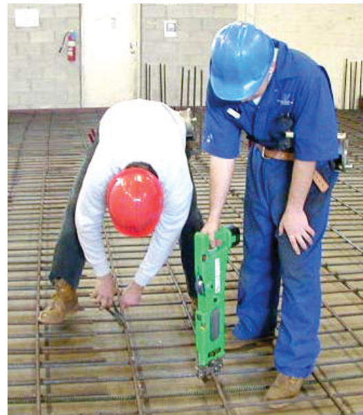
Figure 6: MAX RE-BAR-TIER with arm extension (top) and U-TIER with body extension (bottom). Sometimes a metal hook is used to pull the rebar off the ground so that the wire can be wrapped around the rebar without striking the ground (see top photo).
