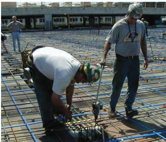
Figure 3: Working posture while working with the rebar tying machine and manually tying rebar.
